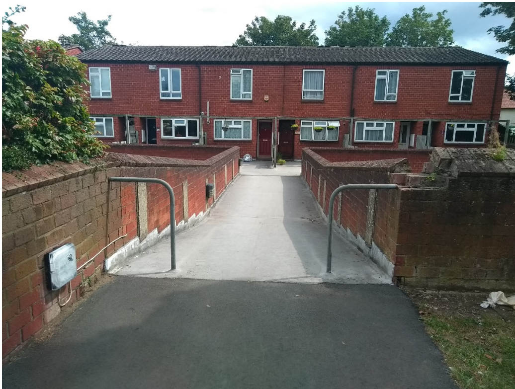
Whitehall Road safety rail installation - Before
